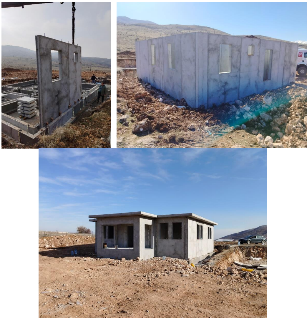
Fig. 1 Precast building constructed using EBM-based construction materials.
